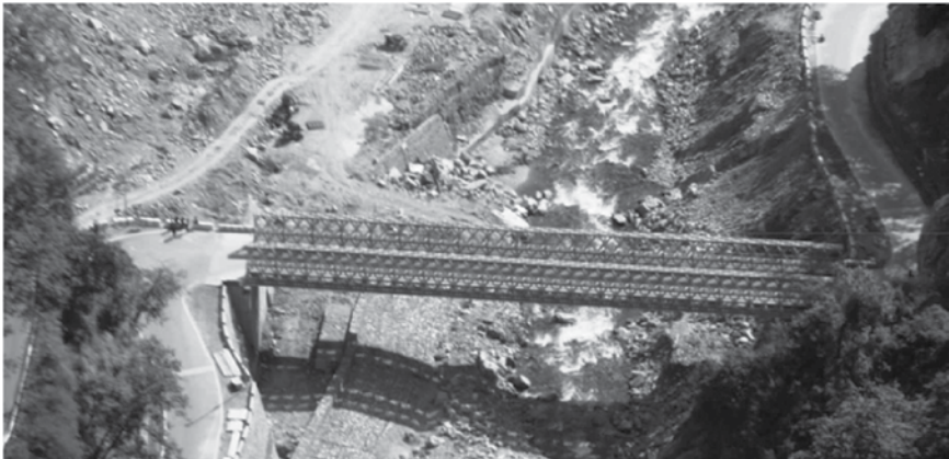
Fig 5: The 60m, double lane, permanent ACROW bridge launched in record time at Sonprayag, en-route to the Kedarnath Shrine (March 2016)
